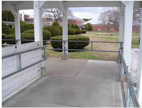
Figure 4: Outdoor walkway (pergola) at MHS lined with metal railings
